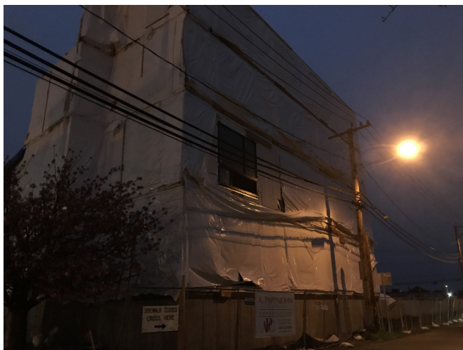
The status of Spinnaker’s Maritime Village on Thursday evening.
